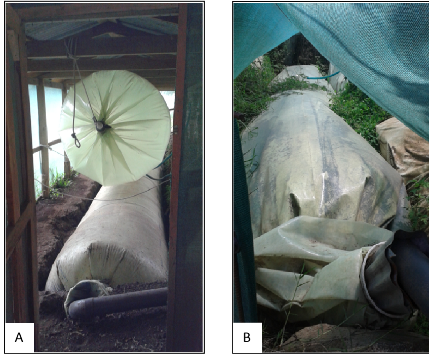
Figure 2.3: Images of tubular digesters with and without a biogas storage bag treating swine waste in Costa Rica
